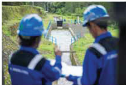
Desand to waterway structure
