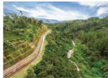
Waterway / Open channel
